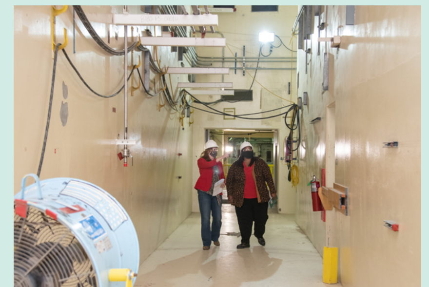
SRPPF Deputy Project Director Rachel Faub (left) and Project Manager April Cox discuss plans for SRPPF, as they walk through the structure that will be repurposed for the pit production mission.
