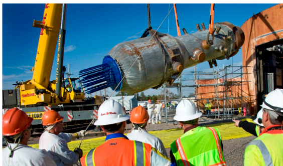
A Recovery Act employee guides the Heavy Water Components Test Reactor (HWCTR)'s 220,000-pound reactor vessel to the ground after removing it from the dome opening.
