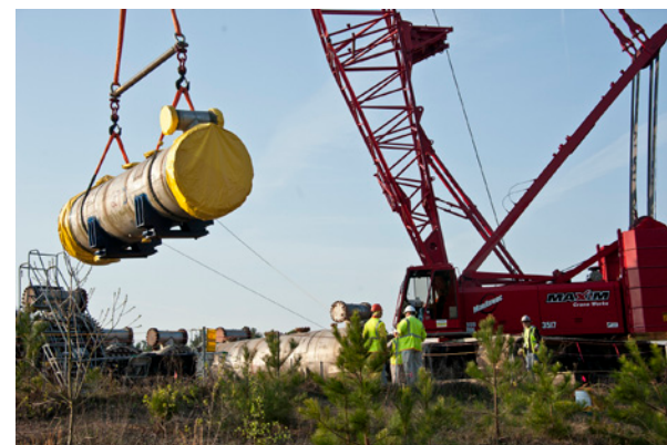
A crane safely lifts a heat exchanger onto a truck trailer.
