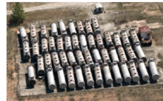
Heat exchangers on the 745-N pad
