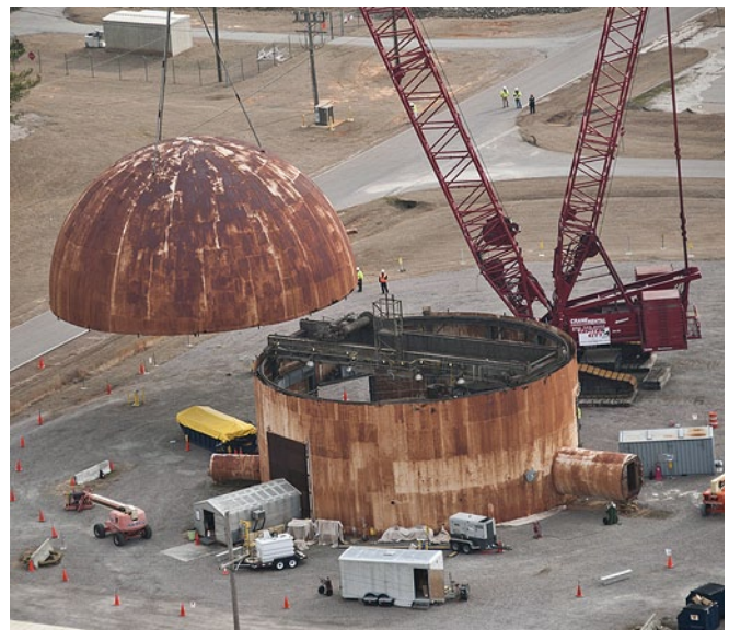
Site ARRA workers achieved the significant milestone of decommissioning the Heavy Water Components Test Reactor, affectionately known as “Hector,” safely removing its rust-orange, 75-foot-tall, 174,000-pound dome with a 660-ton crane and lifting lugs, after more than 16 months of preparations.
