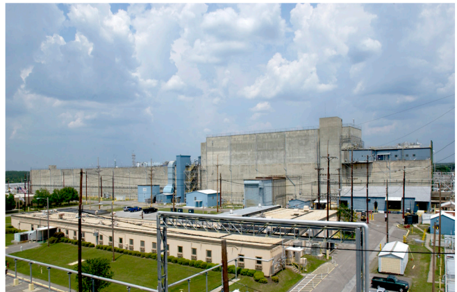
H Canyon at the Savannah River Site
