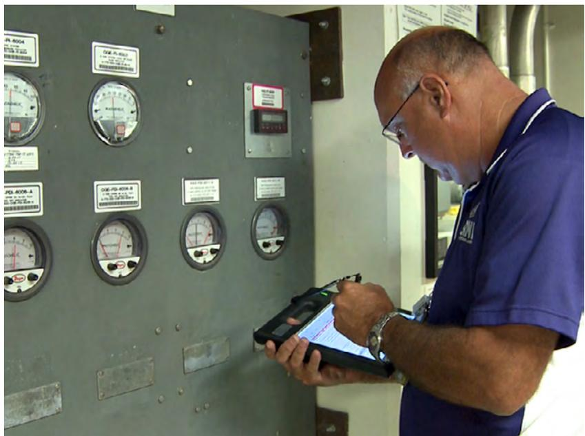
*SRNS employee Matthew Gay uses critical electronic rounds to take a reading at the Savannah River National Lab. Critical electronic rounds, a Continuous Improvement initiative, reduced Operator readings from 326 to 26, freeing up as much as 3.5 hours per shift to work on other facility needs. The validated annual savings are 730 man-hours and over \$42,000.*
