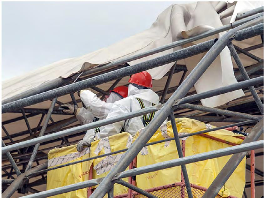
*A former 10,000 square foot waste storage facility at SRS has been completely dismantled. In all, 18,500 square yards of wall and roofing material and 60,000 pounds of steel were removed for permanent disposal.*
