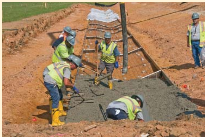
A Recovery Act Project is paving a 3,800-foot long ditch at the H-4 basin, improving drainage and directing the flow of stormwater.
