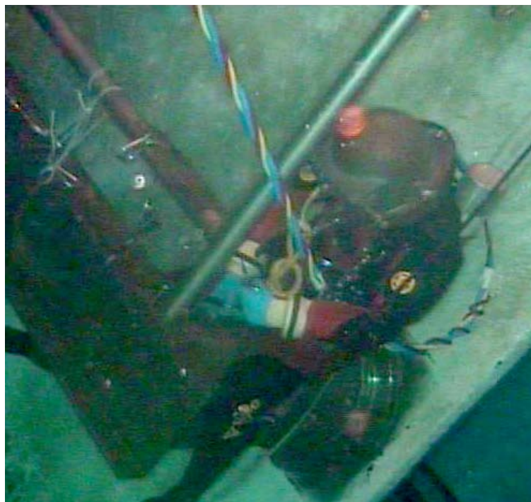
A contracted diver repairs an underwater structure in an L Area Spent Nuclear Fuel storage pool.
