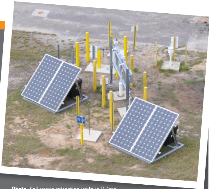
Photo: Soil vapor extraction units in P Area
