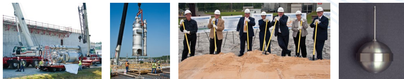
Photos (top): A "topping-out" ceremony was held in 2011 for the WSB | (from left) Giant cranes safely lower an evaporator into the WSB | TRIM groundbreaking at the Tritium Facilities | An example of a tritium reservoir (unclassified) |
