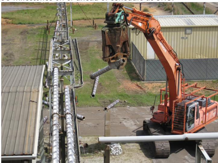
A portion of the 4,000 environmental cleanup milestones met by the Department of Energy and Savannah River Nuclear Solutions (SRNS) over the years involved cleanup of the site's D Area. Here, SRNS personnel manage the demolition of structures and steam lines that crisscrossed this major remediation project.
