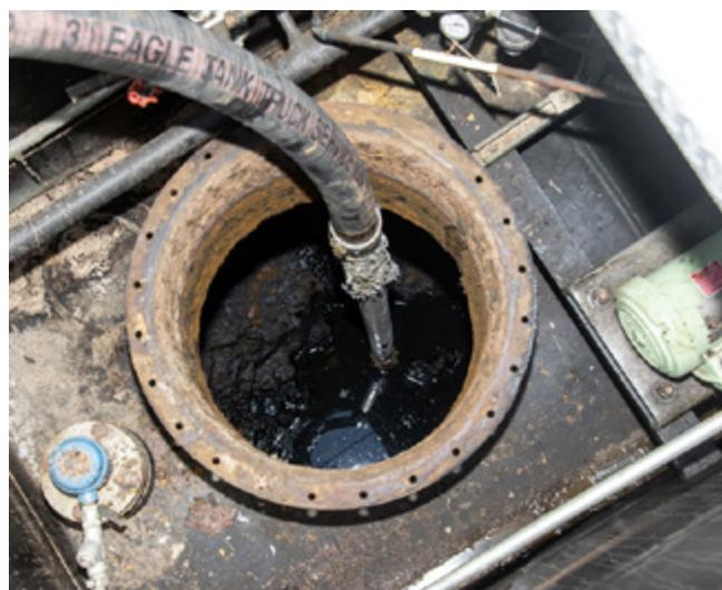
*(right) A special vacuum-equipped truck was used to remove water, exposing a layer of sludge containing silver to be processed and delivered to the U.S. Precious Metals Repository.*
